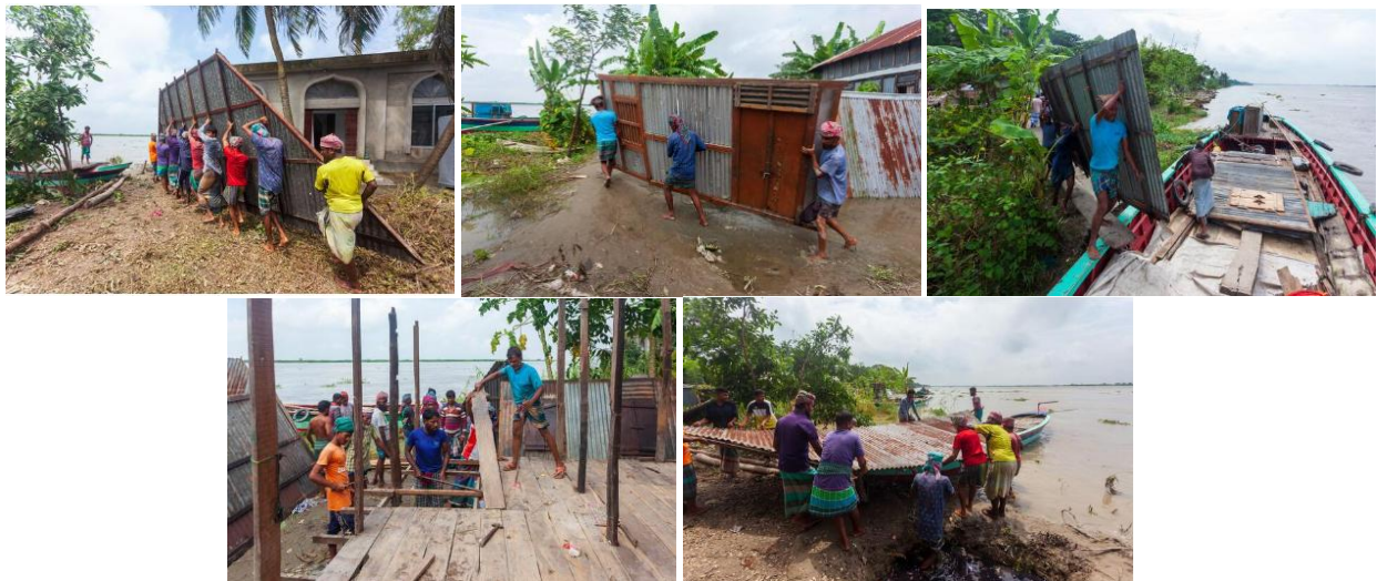
Figure 03. The modular façade panels layer- wooden main frame, galvanized plain sheet, curved wooden planks; Modular houses being shifted in crisis moment (Source: Derived from local news).
