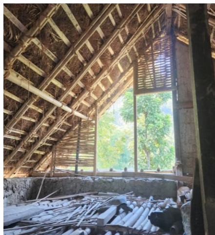
Figure 7. Roof of Mud house.
