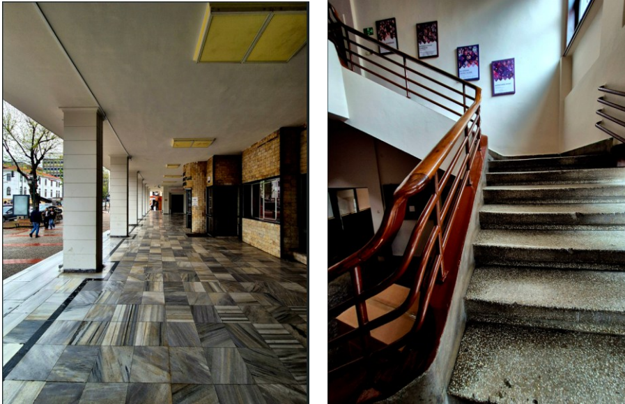
Figure 4. The collonaded entrance hall and the interior details of the Ahmet Vefik Pasha Theater. (Author’s personal archive).
